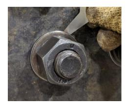
Standard DTIs to be installed and inspected using Feeler Gauge only.
