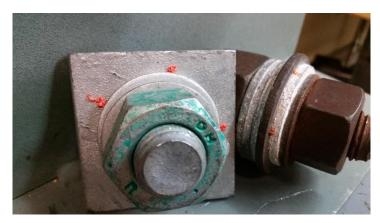
DuraSquirt® DTIs, are enhanced ASTM F9591 DTIs that render feeler gauges unnecessary. Like Squirter® DTIs, DuraSquirt® DTIs expel orange indication media when a bolt has been properly pretensioned in accordance with AISC/RCSC specifications. The difference with DuraSquirt® DTIs, is the indication media is permanent, unless actively removed.
