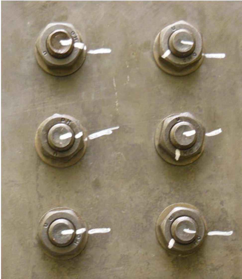
Figure 1: Ideal marking technique clearly indicating 1/3rd turn, However, the three bolts on the left are ready for initial inspection; the three on the right appear turned but it is impossible to know if they were turned or marked to appear turned.
