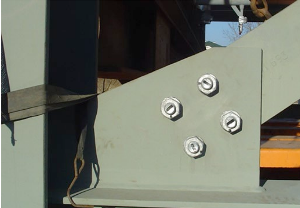
Figure 3: These four nuts appear to have been turned although the exact angle is not obvious since the lines extend completely through the bolts' diameters. Nevertheless, without inspection of their initial position, turn or whether the joint was properly snug-tightened, induced pretension cannot be verified.
